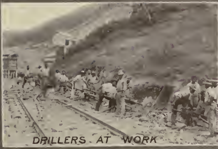
DRILLERS AT WORK
